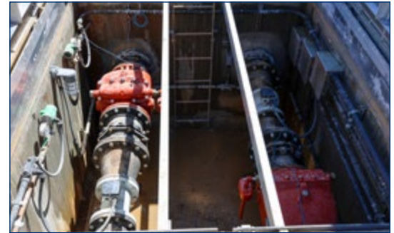
New pipe connection between the two systems
